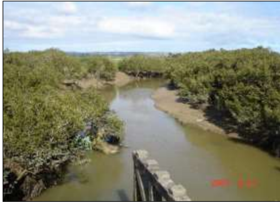
Figure 5-9: Canal, collector drain and minor drain
