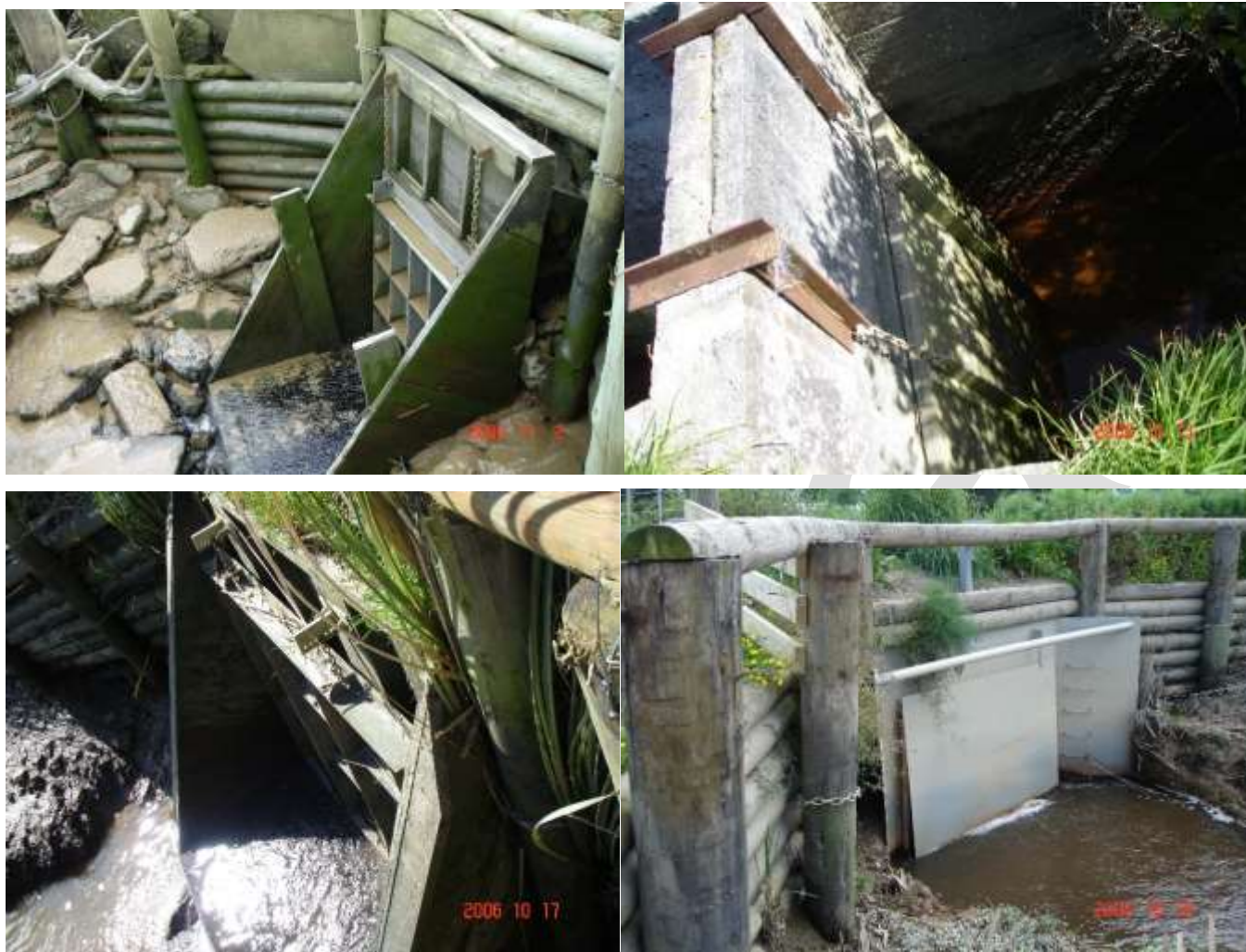
Figure 5-2: Various floodgate types
